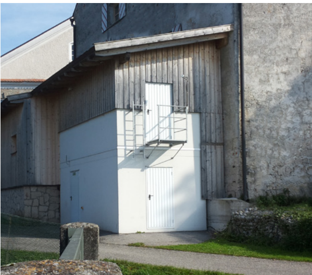
MR Service (Contracting), Schloss Frauenstein, 100 kW Hackgut
