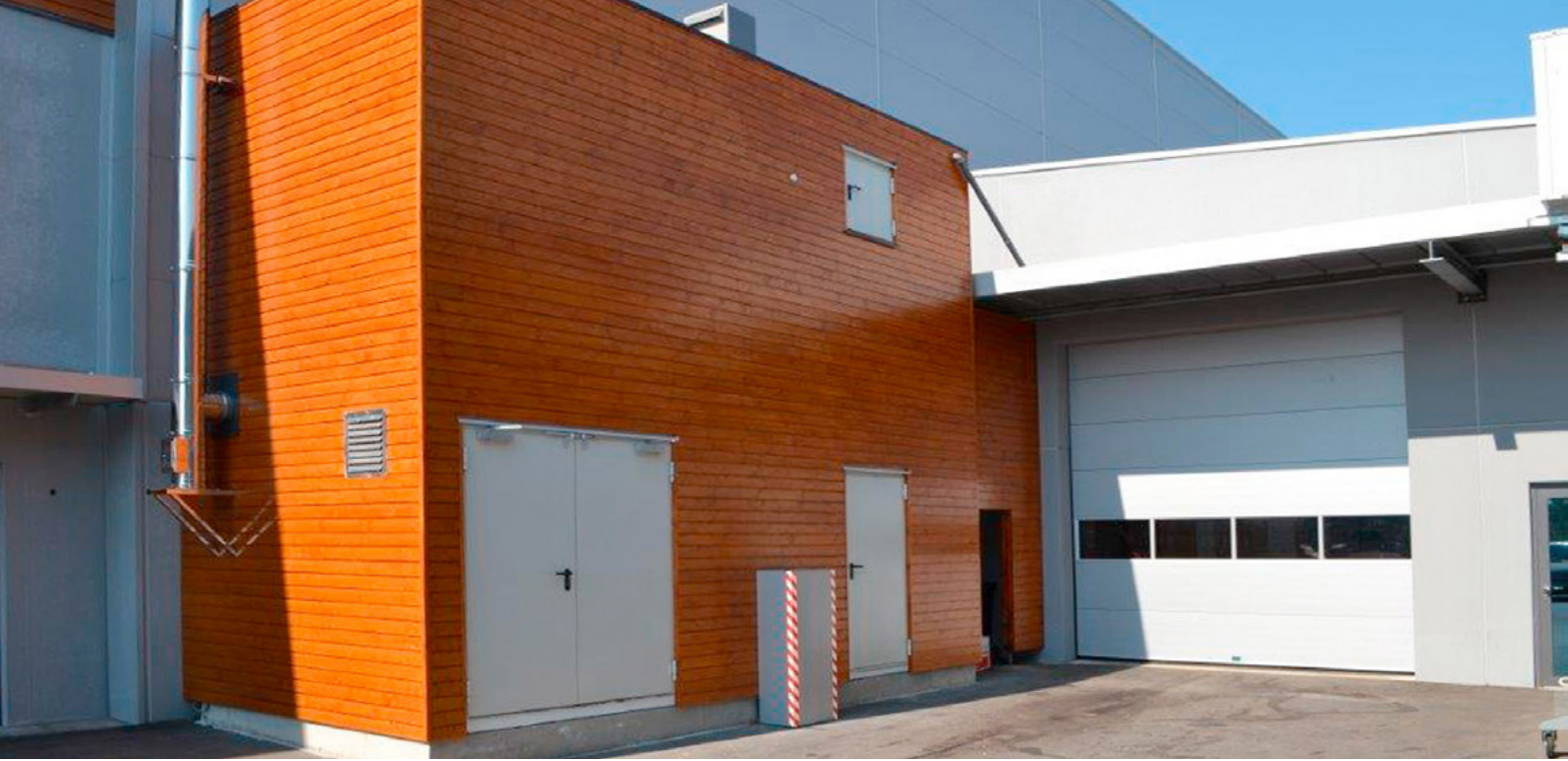
Isana Naturfeinkost in Eresing, 200 kW Hackgut
