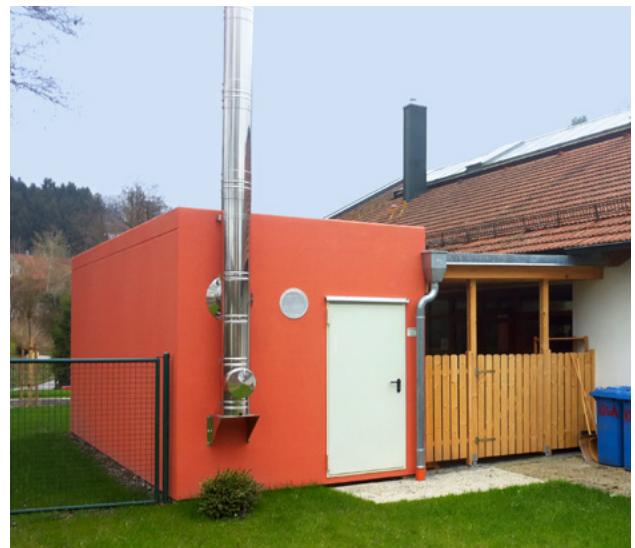
Kindergarten in Windorf, 70 kW Pellets
