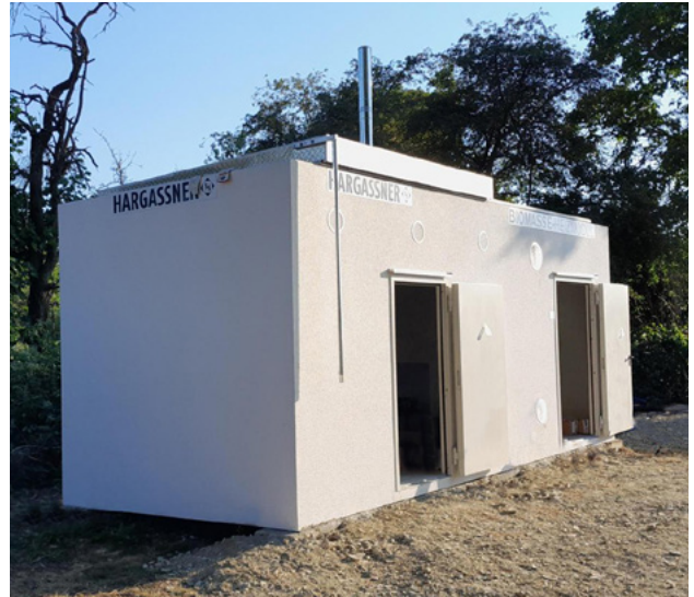
Sonrey in Dransfelden, 40 kW Hackgut
