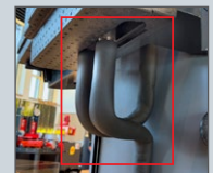
Pipe set for layered accumulator SP with FWS freshwater station
