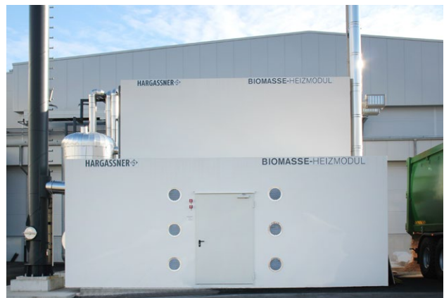
Multiple heating module 660 kW wood chips, industry
